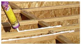
RainBuster 345 Squeak Eliminator is entirely unlike typical subfloor adhesives. Designed specifically to prevent floor squeaks, its innovative technology permanently maintains the sheeting to joist bond. Experience a dramatic reduction in floor squeaks, call back costs and warranty claims by specifying RainBuster 345.
