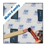
RainBuster 530 offers superior quality and value in a woven building wrap. As part of the RainBuster Leak Free Weatherization System, it functions as a secondary barrier behind exterior cladding, providing protection against water and air infiltration. RainBuster 530 features a woven and coated polyethylene matrix for superior water resistance and strength. In addition, it features a micro-perforated surface, providing vapor permeability to further promote dry wall structures.
